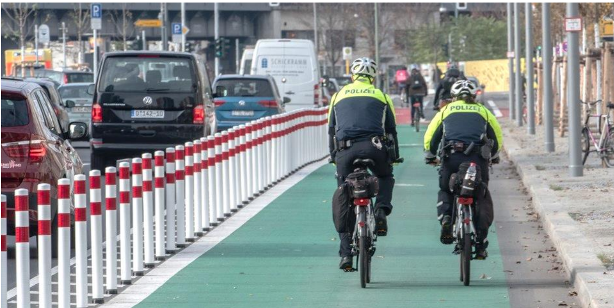
Figure 27 - Protected bike lanes with red and white bollards on Holzmarktstraße in Berlin (Prösser 2018)
